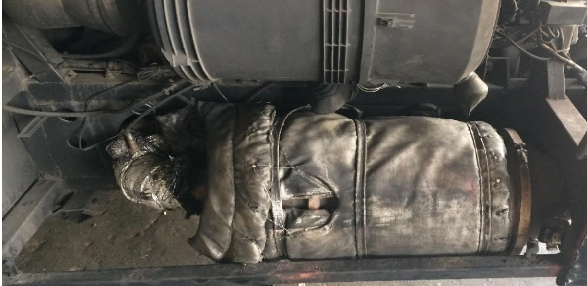
Figure 1. Unsuitable filter isolation
